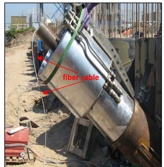
Tensioning of a grout anchor
