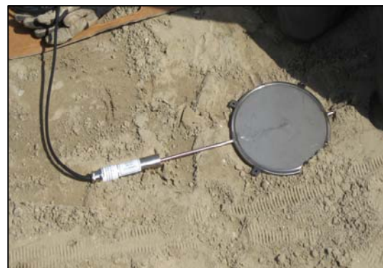
Installation total pressure cells
