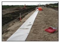
Geotextile with integrated optical fiber
