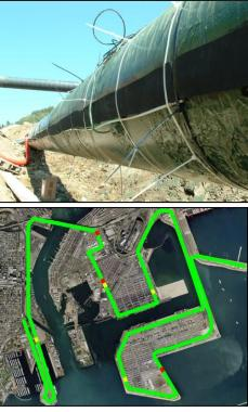
Visualisation of a DSS-system for a pipeline
