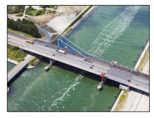
period of two years. The sensors will be interrogated with a frequency of once per hour. During a number of train passages the measurements will take place with an increased frequency of 10 Hz. The measurement data are presented online in real time. The monitoring system will be in operation until the end of 2020.
