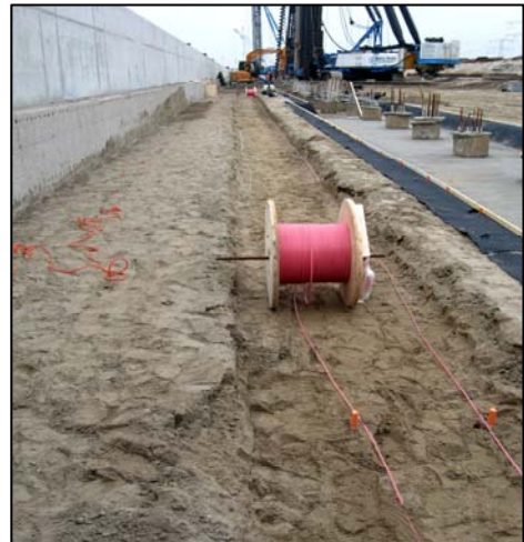
Installation of erosion detection cables
