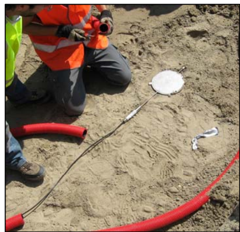
Installation of a total pressure cell
