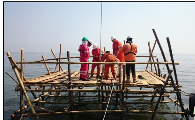
Installation of a SAAF
