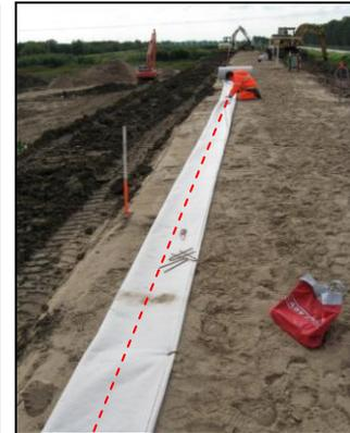
Geotextile with integrated fiber optic cable
