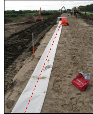
Geotextile with integrated fiber optic cable
