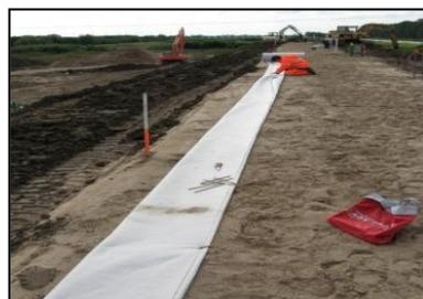
Geotextile with integrated optical fiber
